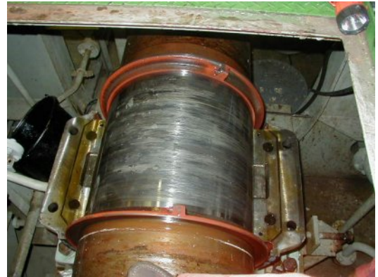
Damaged 505mm Ø Tailshaft Journal
